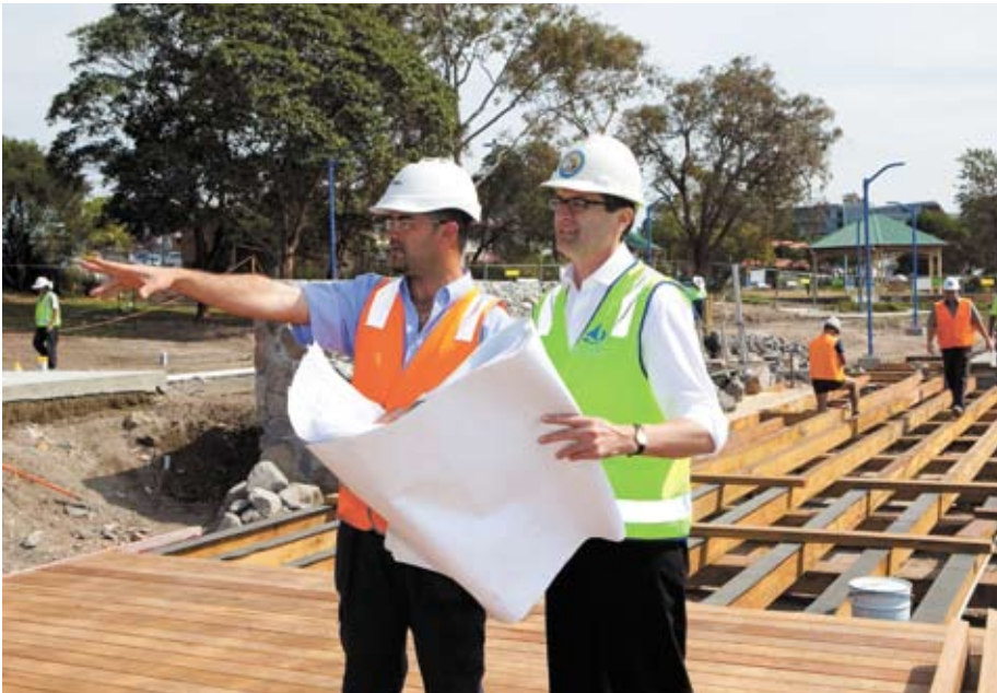
Greg on site with workers at Toronto.
